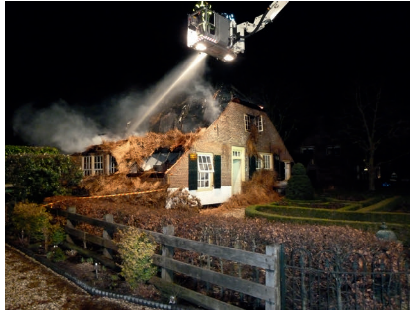
Fire in a monumental farmhouse in the Dutch village Heien Boeicop. Foto: RCE, 2013
