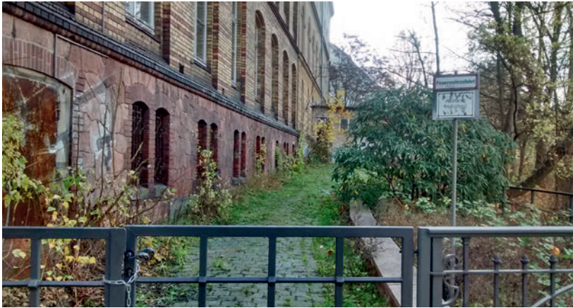
Good accessibility for the fire brigade is very important for heritage! Foto: H. Nuijten/RCE
